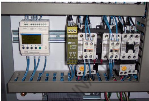
If the phase is correct upon electrical connection the Pilz Phase Sequence Monitor will have a green light on.
