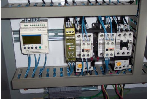
If the Red fault light comes on upon startup, the phase rotation is incorrect and the machine will not operate.
